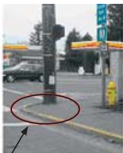
• No Curb Cut
